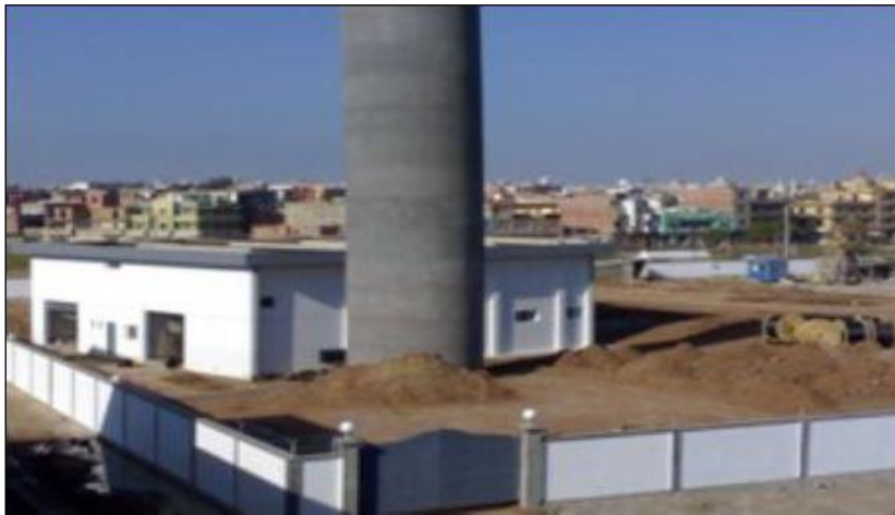
Figure 16. Station de pompage
